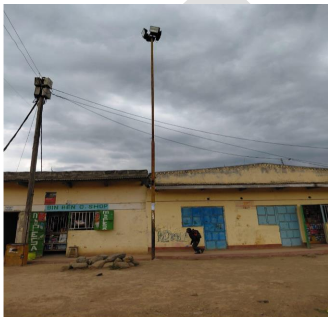
plate 6 - Floodlight at Ngomongo
