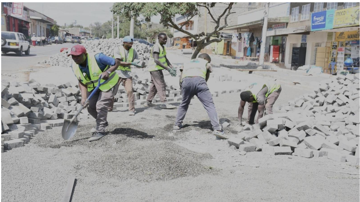
municipal non-motorized transport walkway construction
