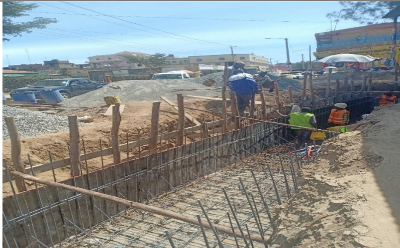
Box culvert Drainage along Mama Ngina Street
