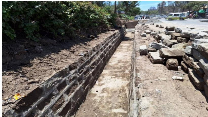
Drainage Constructed along Mama Ngina street
