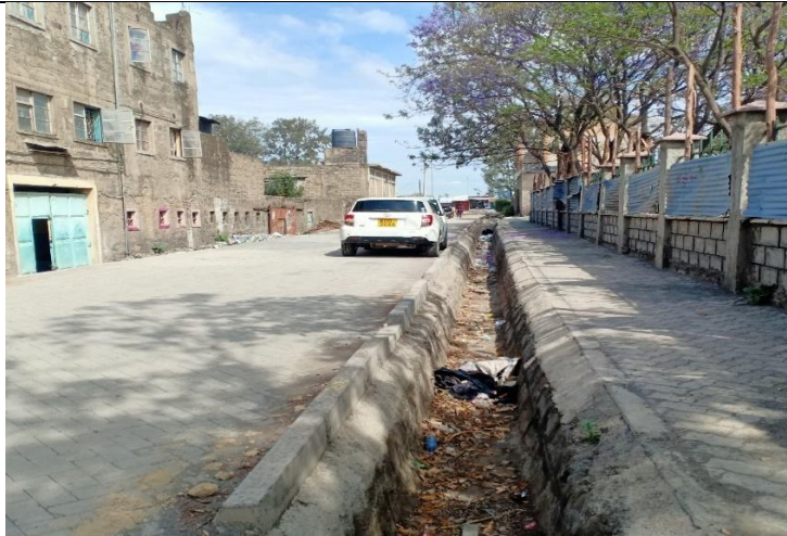
Drainage, Cabro Paving and NMT along adjacent roads to the park
